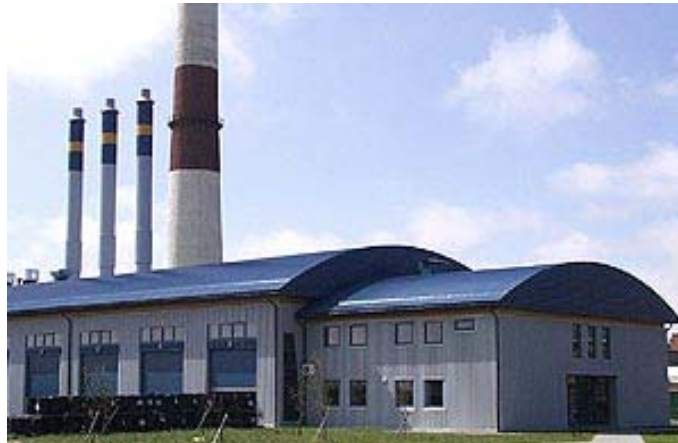
Klaipėda Geothermal plant – general view
